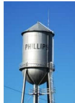
The City of Phillips storage facilities consist of two above ground, elevated tanks or water towers. One water tower is located on Peterson Drive. The above ground tank is able to hold 100,000 gallons of water. The second water tower is located at Balsam Street. The tank can hold 250,000 gallons of water.
